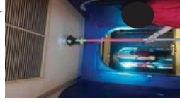
FL24 ROOM 2416 TEST SMOKE DETECTOR 2 HEAD AND HEAT 1 HEAD...NORMAL
