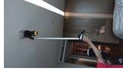
FL21 ROOM 2109 TEST SMOKE DETECTOR 2 HEAD AND HEAT 1 HEAD...NORMAL
