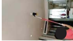
FL 16 Room 1610 Test Smoke detector 1 set and heat 1 set
