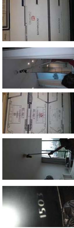
FL28 ROOM 2801 TEST SMOKE DETECTOR 3 HEAD AND HEAT 1 HEAD...NORMAL
