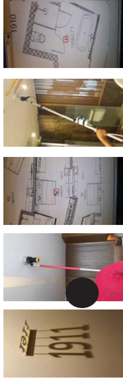
FL19 ROOM 1911 TEST SMOKE DETECTOR 1 HEAD AND HEAT 1 HEAD...NORMAL
