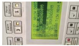
FL 25 Room 2512 Test Smoke detector 2 set and heat 2 set
