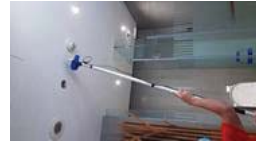
FL 19 Room 1914 Test Smoke detector 1 set and heat 1 set
