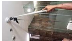
FL18 ROOM 1803 TEST SMOKE DETECTOR 1 HEAD AND HEAT 1 HEAD...NORMAL
