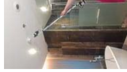
FL24 ROOM 2416 TEST SMOKE DETECTOR 2 HEAD AND HEAT 1 HEAD...NORMAL
