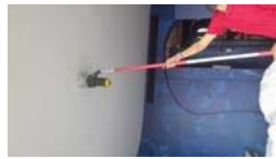
FL21 ROOM 2108 TEST SMOKE DETECTOR 2 HEAD AND HEAT 1 HEAD...NORMAL
