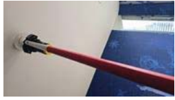
FL 17 Room 1713 Test Smoke detector 1 set and heat 1 set
