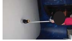
FL21 ROOM 2107 TEST SMOKE DETECTOR 2 HEAD AND HEAT 1 HEAD...NORMAL
