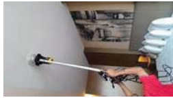
FL17 ROOM 1717 TEST SMOKE DETECTOR 1 HEAD AND HEAT 1 HEAD...NORMAL
