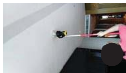
FL 20 Room 2001 Test Smoke detector 1 set and heat 2 set
