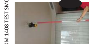
FL14 ROOM 1405 TEST SMOKE DETECTOR 1 HEAD AND HEAT 1 HEAD...NORMAL
