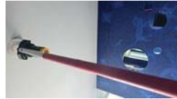
FL 24 Room 2415 Test Smoke detector 2 set and heat 1 set
