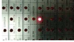
FL 25 Room 2505 Test Smoke detector 2 set and heat 2 set
