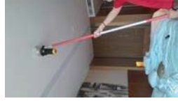
FL19 ROOM 1918 TEST SMOKE DETECTOR 1 HEAD .. NOWORK AND HEAT 1 HEAD...NORMAL
