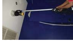
FL27 ROOM 2706 TEST SMOKE DETECTOR 1 HEAD AND HEAT 2 HEAD...NORMAL
