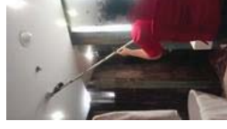
FL19 ROOM 1918 TEST SMOKE DETECTOR 1 HEAD .. NOWORK AND HEAT 1 HEAD...NORMAL
