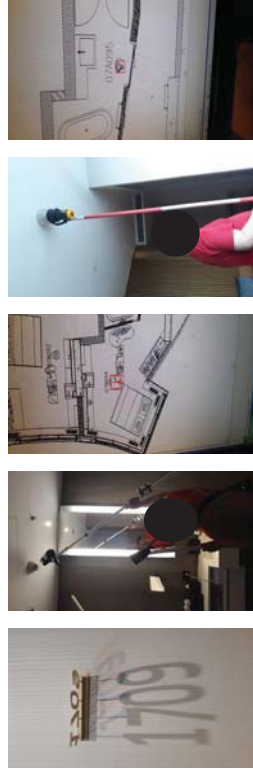
FL18 ROOM 1810 TEST SMOKE DETECTOR 1 HEAD AND HEAT 1 HEAD...NORMAL
