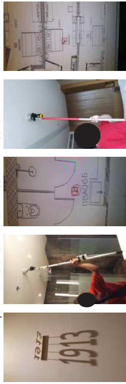
FL19 ROOM 1913 TEST SMOKE DETECTOR 1 HEAD AND HEAT 1 HEAD...NORMAL
