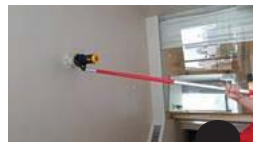
FL 24 Room 2406 Test Smoke detector 2 set and heat 1 set
