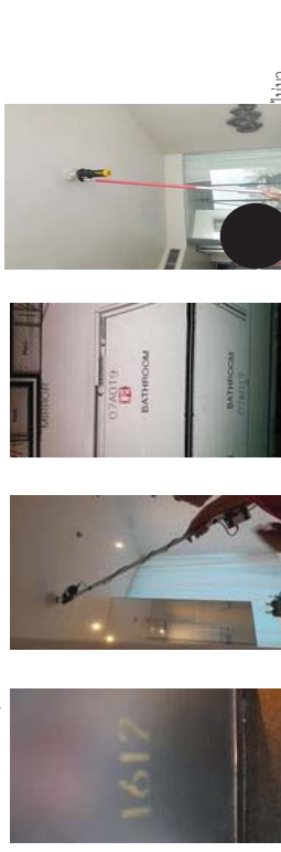
FL16 ROOM 1617 TEST SMOKE DETECTOR 1 HEAD..NOWORK AND HEAT 1 HEAD...NORMAL
