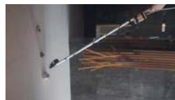
FL19 ROOM 1907 TEST SMOKE DETECTOR 1 HEAD AND HEAT 1 HEAD...NORMAL
