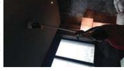
FL27 ROOM 2706 TEST SMOKE DETECTOR 1 HEAD AND HEAT 2 HEAD...NORMAL
