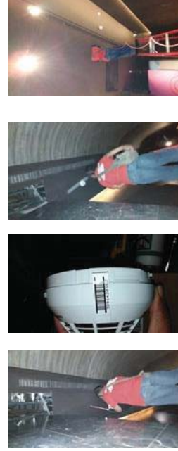
FL 16 Room 1613 Test Smoke detector 1 set and heat 1 set
