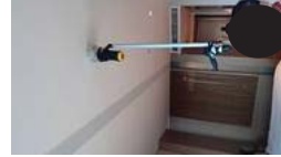
FL18 ROOM 1806 TEST SMOKE DETECTOR 1 HEAD AND HEAT 1 HEAD...NORMAL
