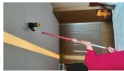
FL19 ROOM 1907 TEST SMOKE DETECTOR 1 HEAD AND HEAT 1 HEAD...NORMAL
