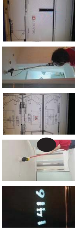
FL14 ROOM 1415 TEST SMOKE DETECTOR 1 HEAD AND HEAT 1 HEAD...NORMAL
