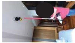
FL 18 Room 1812 Test Smoke detector 1 set and heat 1 set
