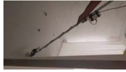
FL16 ROOM 1618 TEST SMOKE DETECTOR 1 HEAD AND HEAT 1 HEAD...NORMAL
