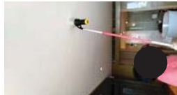
FL 20 Room 2009 Test Smoke detector 1 set and heat 1 set
