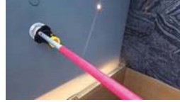
FL 25 Room 2510 Test Smoke detector 2 set and heat 2 set
