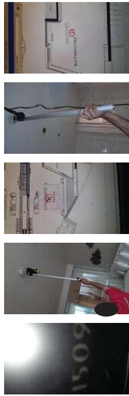
FL15 ROOM 1503 TEST SMOKE DETECTOR 1 HEAD AND HEAT 1 HEAD...NORMAL
