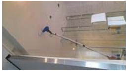
FL 14 Room 1407 Test Smoke detector 1 set and heat 1 set
