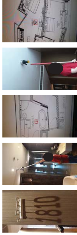
FL19 ROOM 1901 TEST SMOKE DETECTOR 1 HEAD AND HEAT 1 HEAD...NORMAL
