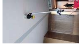
FL18 ROOM 1803 TEST SMOKE DETECTOR 1 HEAD AND HEAT 1 HEAD...NORMAL
