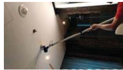
FL 18 Room 1812 Test Smoke detector 1 set and heat 1 set
