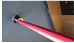
FL 25 Room 2505 Test Smoke detector 2 set and heat 2 set
